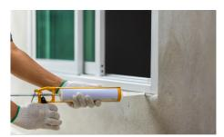
Seal air leaks. While old windows are often characterized as energy losers, it is usually the air leaks around and through them that causes the greatest energy losses. Worn out frames and cracked seals can allow warm air to escape during the winter. Cracked caulking and improper sealing during investigate.
